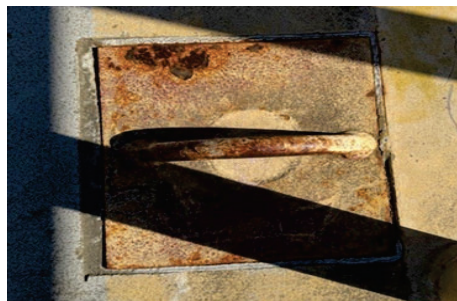
Above, HRST anchor load point. (U.S. Marine Corps photo by GySgt Patrick Doody)
